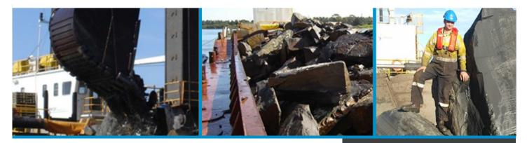
The backhoe dredge Machiavelli, along with 2 x 750m<sup>3</sup> and 2 x 500m<sup>3</sup> hopper barges and tugs Kurutai, Kotor and Nautilus were contracted to dredge 570,000m<sup>3</sup> of marine sediments, stiff clays and rock from the Hunter River for the new Kooragang Berth K10 for Newcastle Coal Infrastructure Group.
