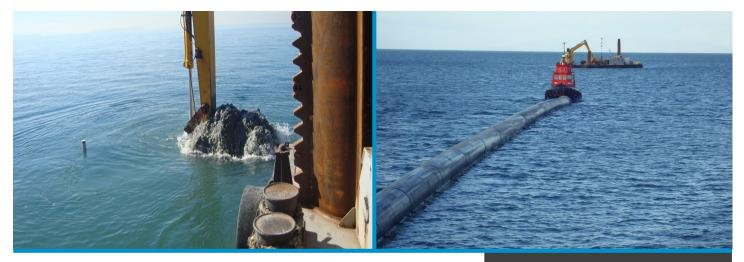
To protect and improve the quality of Auckland's beaches, a new tunnel and outfall was constructed allowing treated water from the Rosedale Wastewater Treatment Plant to be discharged 2.7 kilometres offshore into the Hauraki Gulf.
